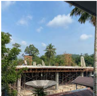
New ward under construction (photo as of July 2025)
